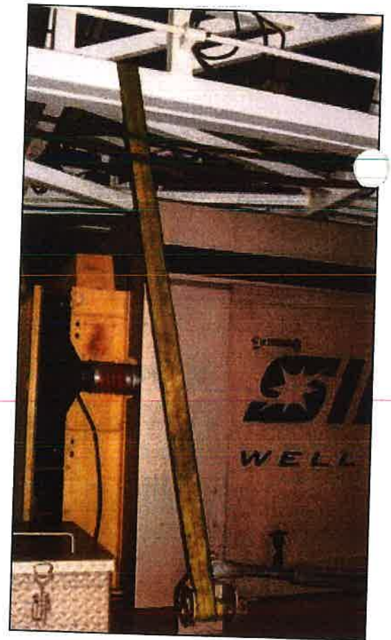
Strapping derrick to carrier
