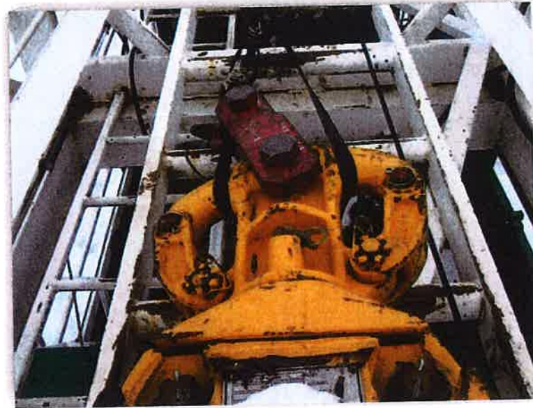
Securing the bottom block
